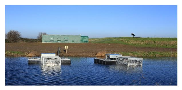
Quality of water coming into the system is monitored by a 7-way sonde that allows a range of water quality parameters to be monitored and the pumps to be stopped if thresholds are reached. Because of the proximity to the sea the biggest concern is saltwater ingress. However, the only concerns to date, have come from elevated conductivity levels related to salt that is spread on the roads during icy conditions, making its way into the drainage water.
