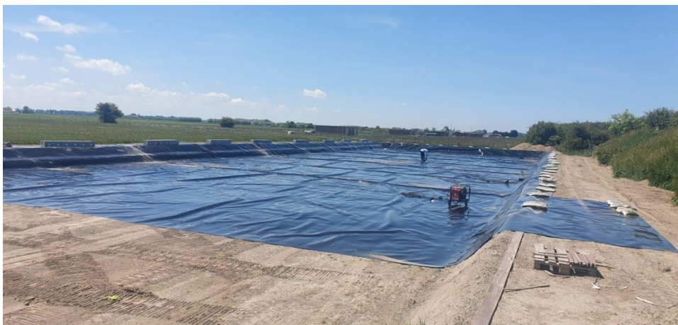
Photo 1. Placement of an impermeable layer at the bottom of the willow marsh
