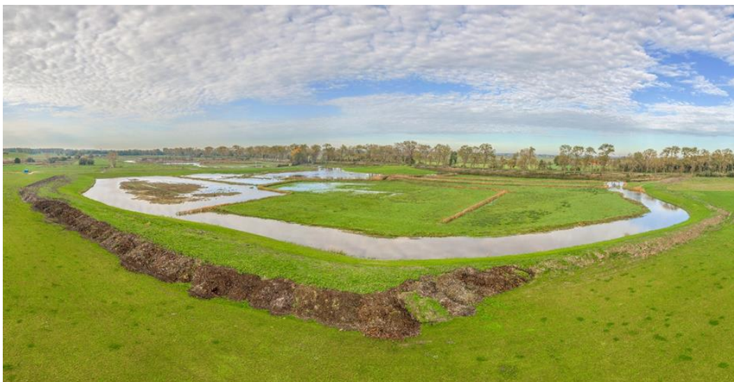
Photo 2 Demo site during filling October 2022. Water level is 1,90 m TAW. At maximum level of 2,40 m TAW, apart from a few islands the entire area will be flooded.
